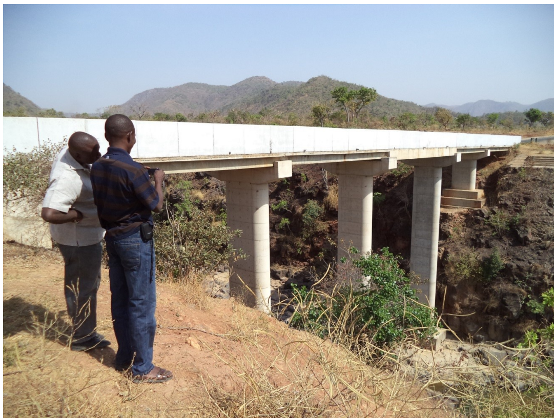
Fig. 12 Jibang Bridge, Quan Pan abutting basalt flows from the Pankshin Hills Central Nigeria
