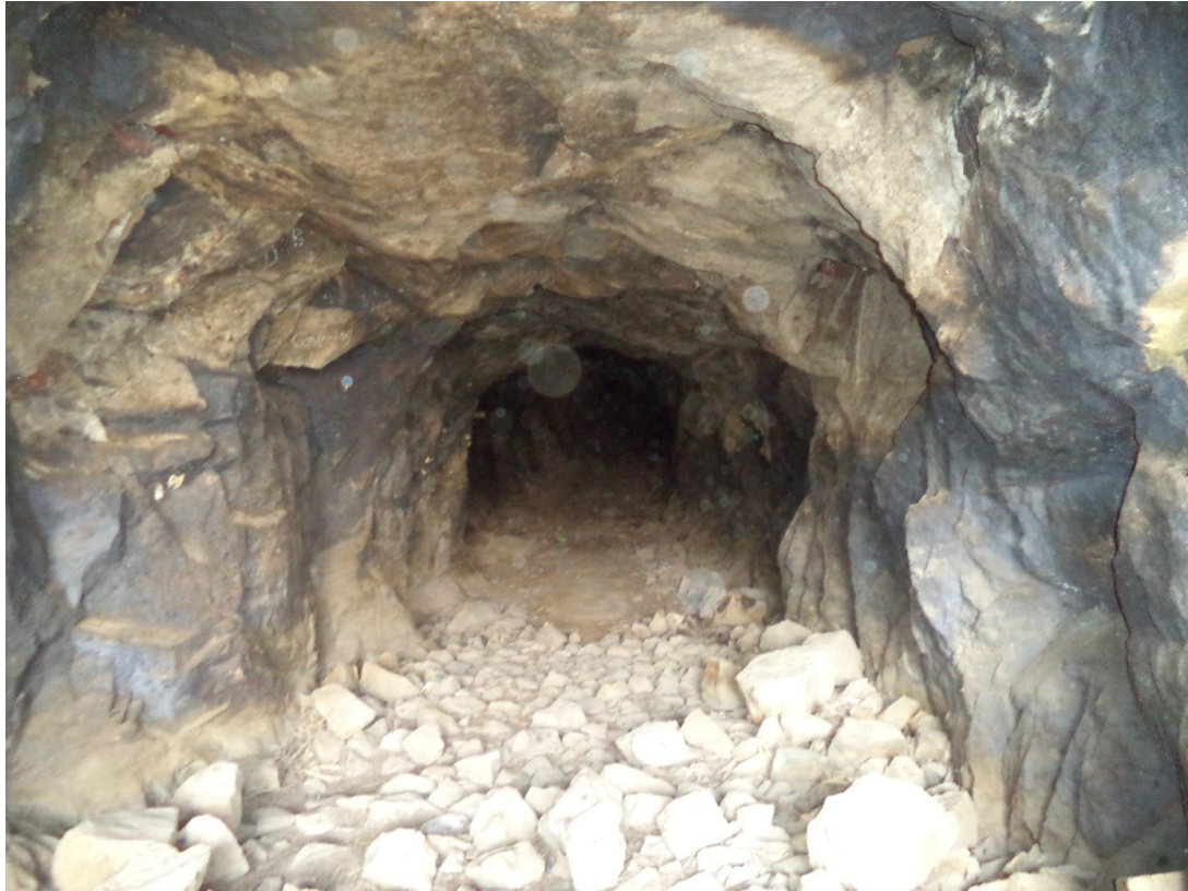
Fig. 15 Naturally stabilized abandoned molybdenite mined out shaft in Kigom Younger Granite Complex, Jos
