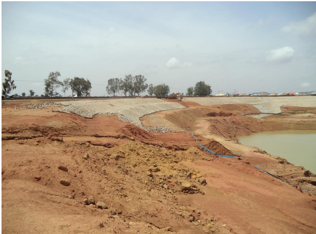
Fig. 2 Photograph showing an attempt to artificially stabilize a pond around Yelwa Club Bukuru.
