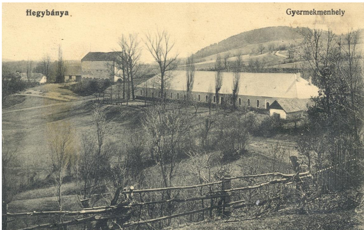
Fig. 6 A view on premises of water pumping devices on the left. (source: Herčko)
